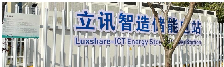
Energy Storage Power Station of Luxshare Smart Manufacturing
