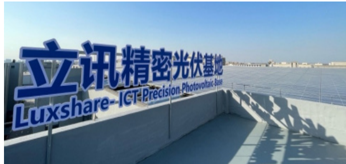
Distributed Photovoltaic Project of Luxshare Smart Manufacturing
